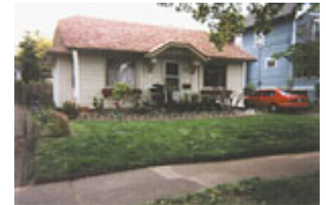
Beth and Zachs 900 sq ft bungalow before the remodel started.
