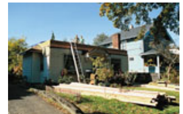
With the roof completely removed next phase second story begins.
