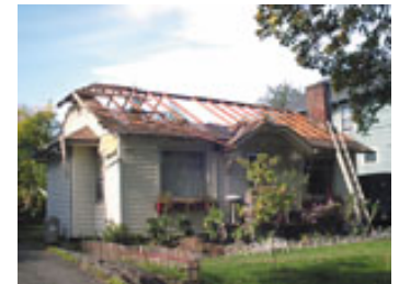
De-construction started with the removal of the roof.
