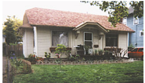
Before construction began on Zach and Beth's, 900 sq ft bungalow.
