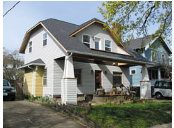
Exterior construction complete except for the finishing touches on the second-story veranda.
